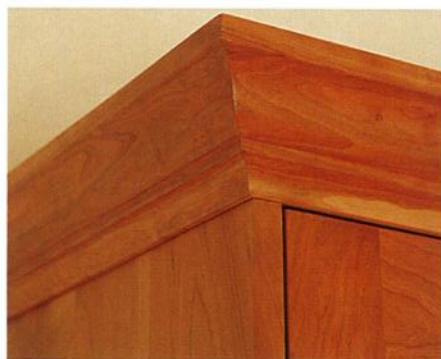
One simple but effective way to finish the top of a wall cabinet is to add crown moulding. The moulding adds a flair to the top, and it gives the cabinet depth as you look up at it. Dentil moulding underneath the crown can add even more flair.
